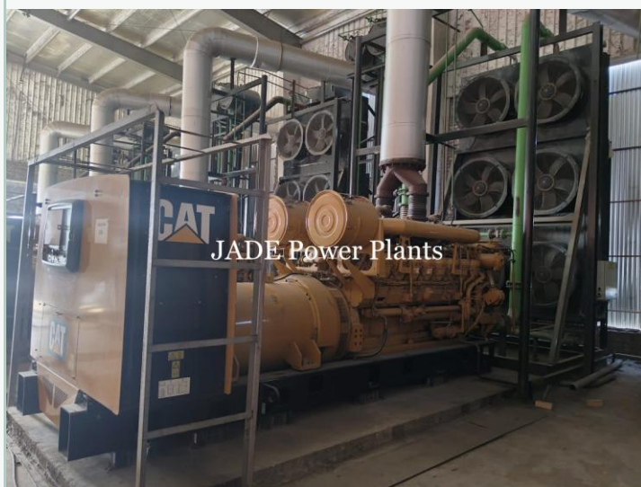
Representative CAT 3516B Radiator-Side View
